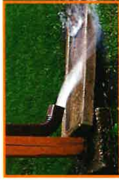
Downspout discharging into yard
